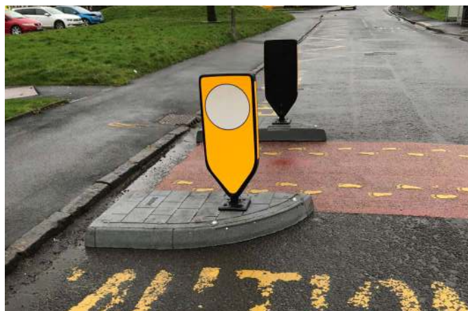
Build outs installed in the location of the street kit
